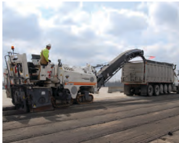
Milling machine milling asphalt road and loading debris into haul truck.
