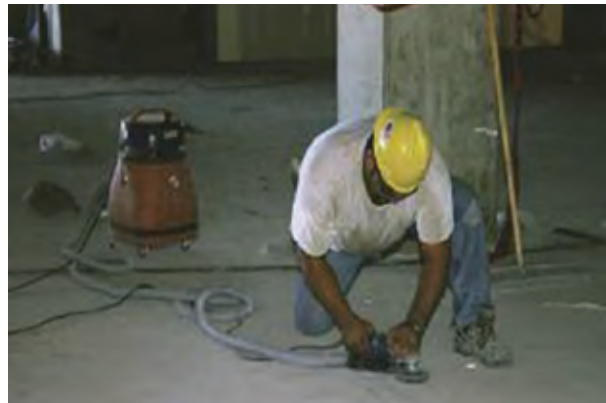
Worker grinding concrete floor with grinder attached to dust collector (background).
