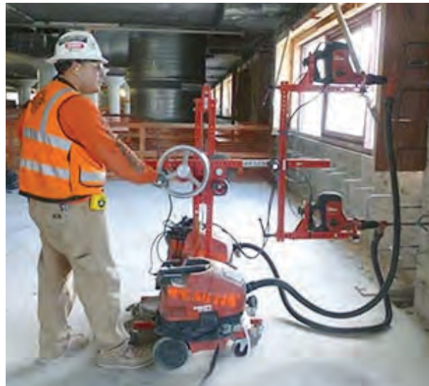
Worker is drilling horizontal holes in a concrete wall using two stand-mounted drills, each equipped with a dust collector. Note the shrouds around drill bits, black hose, and dust collector are attached to the stand.
