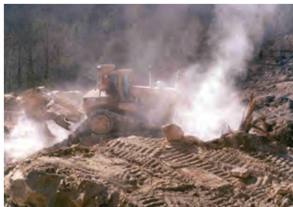
Earthmoving using a dozer equipped with enclosed operator cab.
