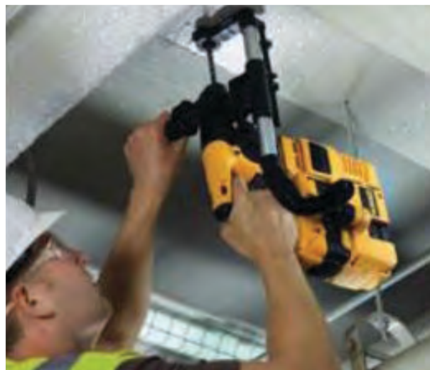
Worker drilling into concrete with a rotary hammer equipped with shroud and dust collection system. Note the shroud around drill bit, silver and black hose, and dust collector are attached conveniently to the drill.
