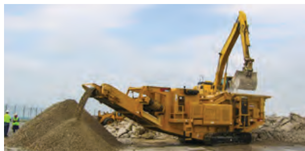
Crushing machine being loaded with construction debris by an excavator
